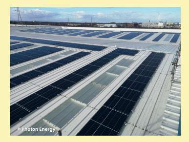
installation team had to complete a thorough site induction before being allowed on the site and a daily permit to work system was in force for both general works and additionally for roof works. The final connection of the PV system to the main electrical panel board was done out of hours on a Saturday as the main board had to be shutdown for safety reasons.
